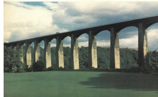
Built in 1805, the Pont Cysylltau Aqueduct extends a canal 1,000 feet across a Welsh valley.
