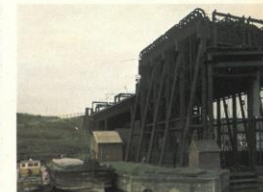
A later development, the Anderton boat lift still raises yachts 50 feet from one canal to another.
